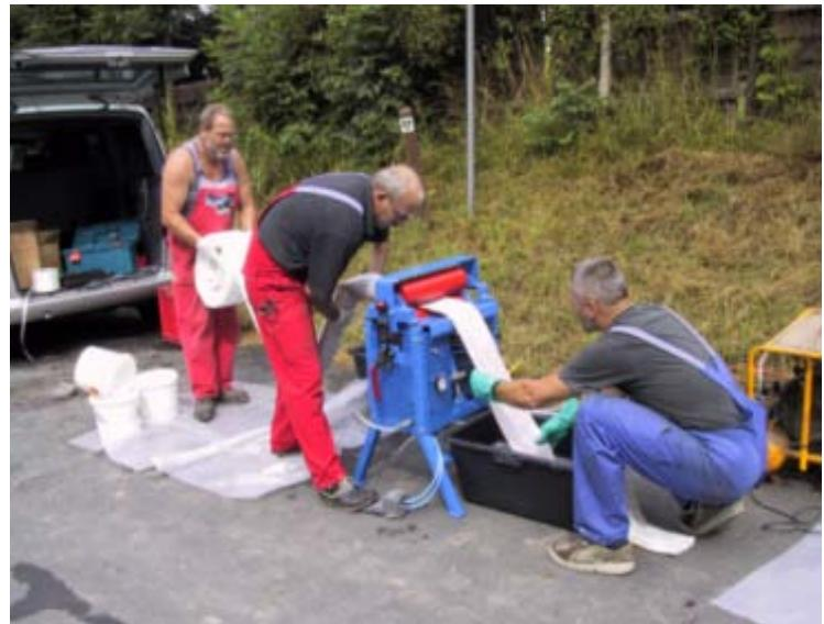
Once all milling work has finished and the drain cleaned, the next step in modern sanitation can be taken. A liner hose is cut to the correct length of the section of drain which needs clearing by the PL-Inliner system of Bodenbender GmbH. It features a needle felt weave and is externally coated with a PVC layer. The hose section is filled with CombiTec epoxy resin on-site and run through an impregnation table so that it is evenly spread out.
