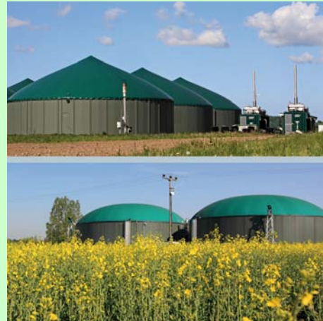
Application examples - biogas plants and CO-generation plants
