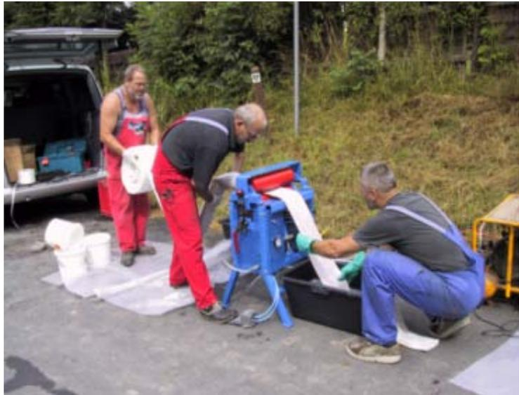
Once all milling work has finished and the drain cleaned, the next step in modern sanitation can be taken. A liner hose is cut to the correct length of the section of drain which needs clearing by the PL-Inliner system of Bodenbender GmbH. It features a needled felt weave and is externally coated with a PVC layer. The hose section is filled with CombiTec epoxy resin on-site and run through an impregnation table so that it is evenly spread out.
